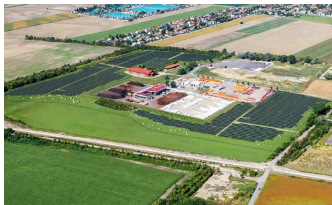
The largest solar power plant in Austria.
