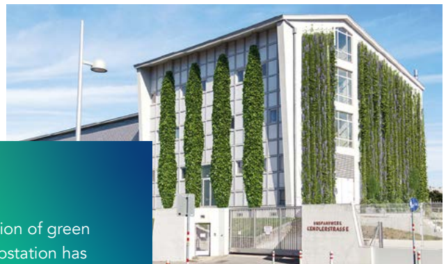
Wiener Netze also creates green views and exteriors.
